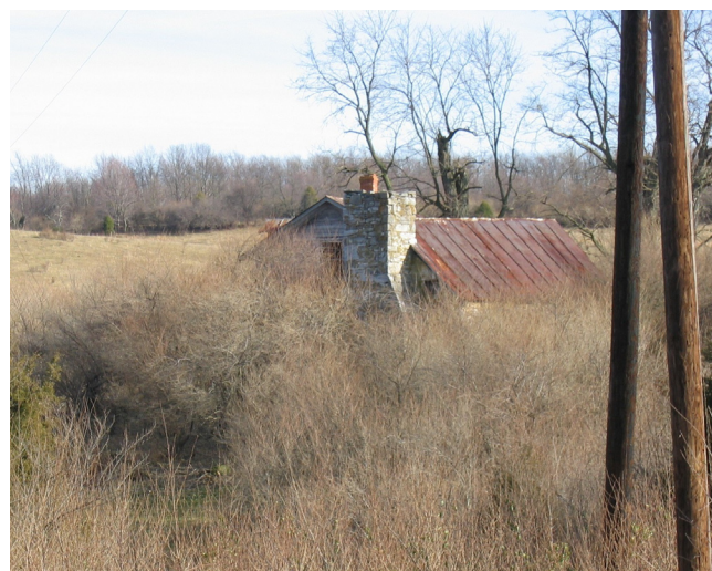
Autumn olive almost engulfing a structure
