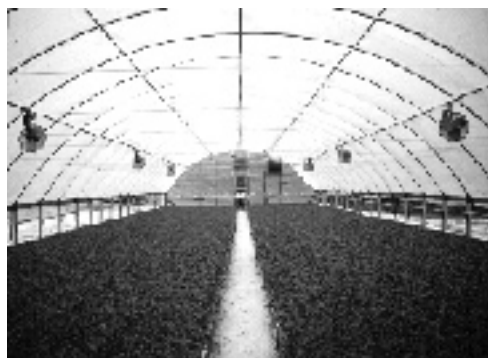
Figure 1. Positioning of horizontal airflow fans (HAF) for air circulation within the greenhouse and the use of side curtains for ventilations
