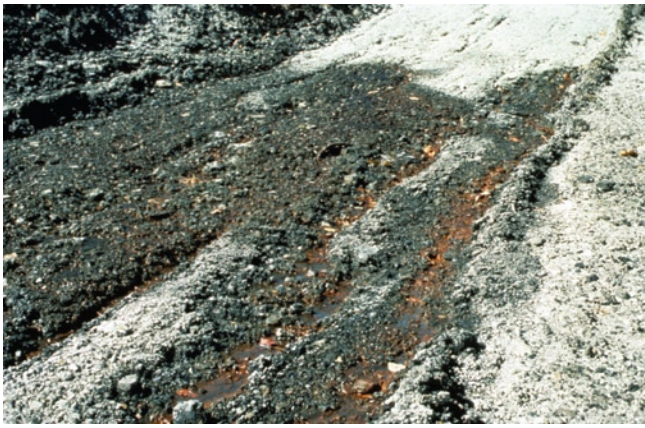
Figure 3. Sulfate salts weeping from an active coal refuse pile. These salts are the product of the acid sulfate weathering process within the fill and are transported to the fill surface by acidified seepage. When the seepage dries at the pile surface, the salts precipitate as seen here. The red colors are evidence of iron that is being released by pyrite oxidation and brought to the surface along with acidic seepage waters.
