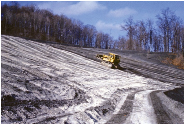
Figure 7. Agricultural limestone being applied and tracked into a coal refuse fill face. Working lime and other amendments on the steeper slopes that dominate most refuse piles can be challenging. For extremely acidic refuse materials, several applications of lime split several months apart may be necessary. It is difficult to spread and incorporate more than 25 tons of lime per acre in one application, even on flat sites.
