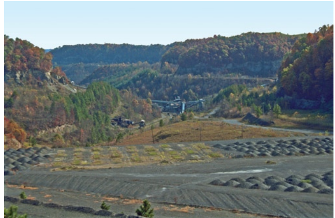
Figure 6. The refuse revegetation guidelines in this publication were developed through methods that included plot-scale field trials, such as those shown in the mid-to-lower left of this photograph, and operational-scale trials conducted by mining firms.
