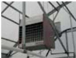
Generally, heater issues (improper installation, cracked heat exchanger, chronic use of unvented heater, leaking gas lines, and improper flame adjustment) can cause ethylene exposure. With fall just around the corner, this is a good time to start thinking about heater maintenance and start-up. Keeping the heating system in good repair and operating condition will not only lessen the chance of ethylene exposure,
