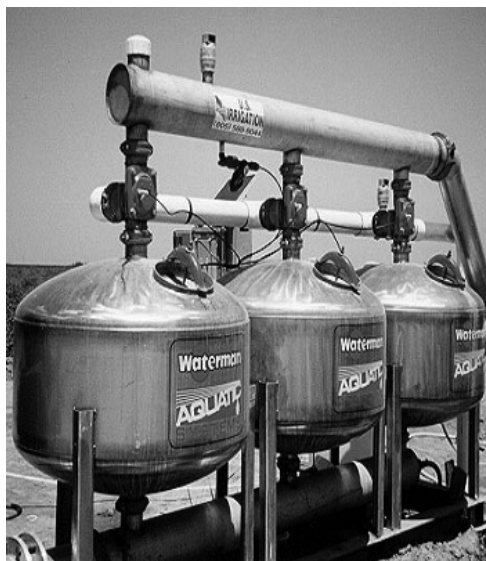
Figure 4. Photo and schematic of sand media filter (photo courtesy of Waterman Industries, schematic adapted from Claude Laval Corp.).
