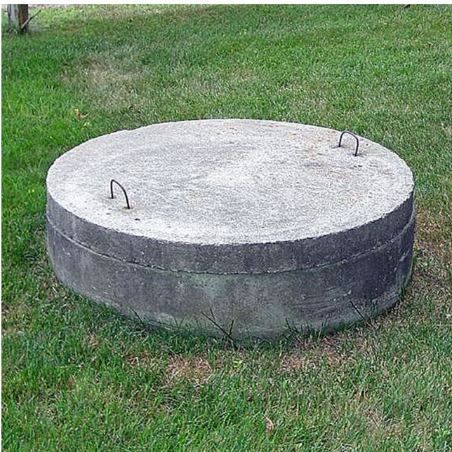
Figure 1b. A bored well with a tightly fitted concrete cap. Source: Bryan Swistock, Penn State University.
