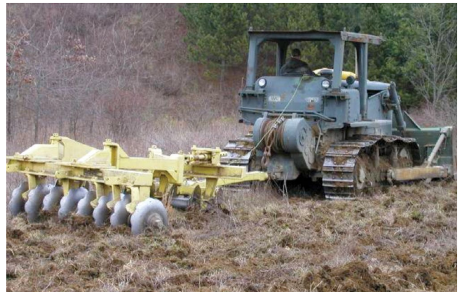
Figure 8. A large disk being used to break up surface soil and herbaceous vegetation root mass prior to soil ripping. This operation is not always necessary, but it can increase the efficiency of the deep tillage operation on sites where dense vegetation is present.
