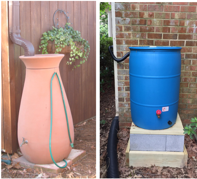
Figure 1. Left, rain barrel connected directly to a downspout; right: rain barrel connected to a downspout with a diverter hose. Photos by L. Fox and Nina Page, Virginia Beach Master Gardner Water Steward.
