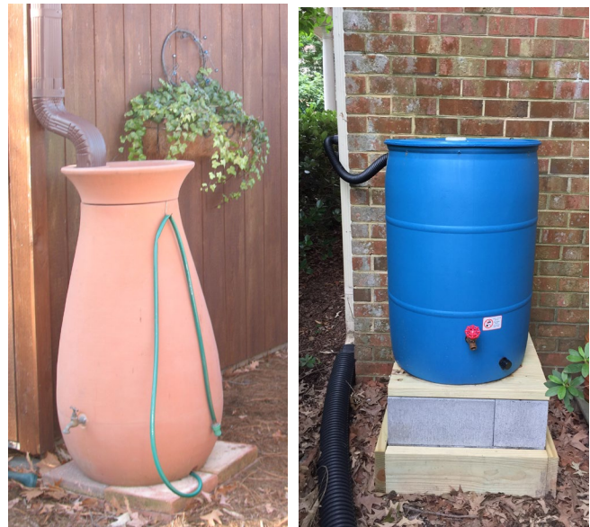
Figure 1. Left, rain barrel connected directly to a downspout; right: rain barrel connected to a downspout with a diverter hose. Photos by L. Fox and Nina Page, Virginia Beach Master Gardner Water Steward.
